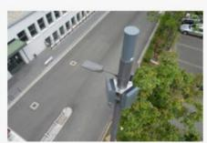
The pole conceals the macro radios delivering 1800 and 2600 MHz in the podium sections of the pole. The Alpha Wireless AW3833-5 cannister antenna is mounted on top of the pole in the same color as the pole. In this installation, G and G Stadtsysteme intentionally used 3.5 GHz antennas to better understand the frequency band.
